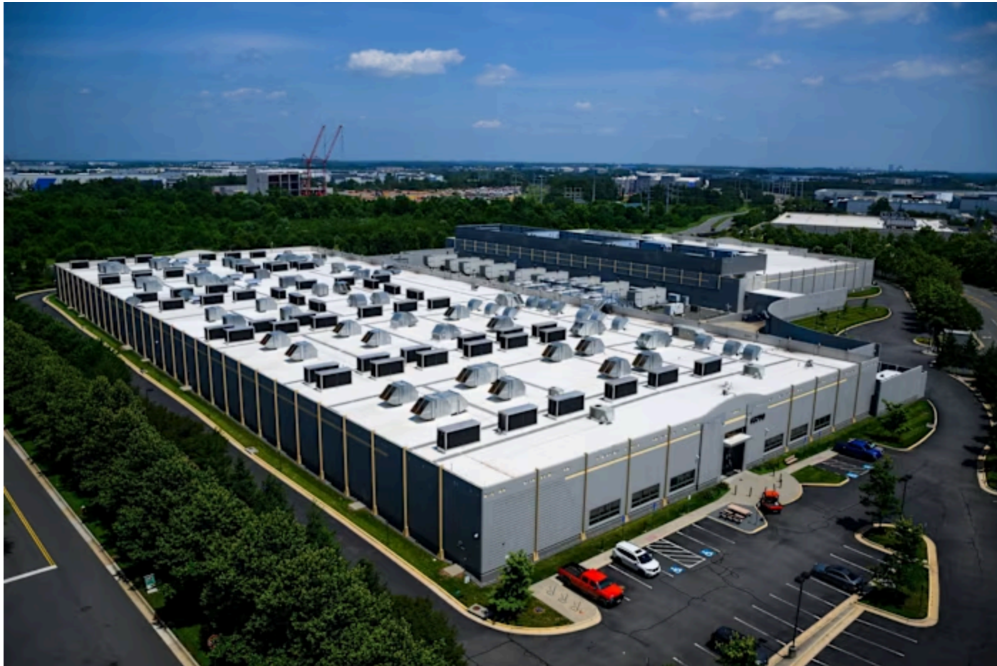
'Data centre alley', a Virginia hub through which almost three-quarters of global search traffic travels. Some locals blame politicians for approving energy-hungry centres © Pete Kiehart/Bloomberg
